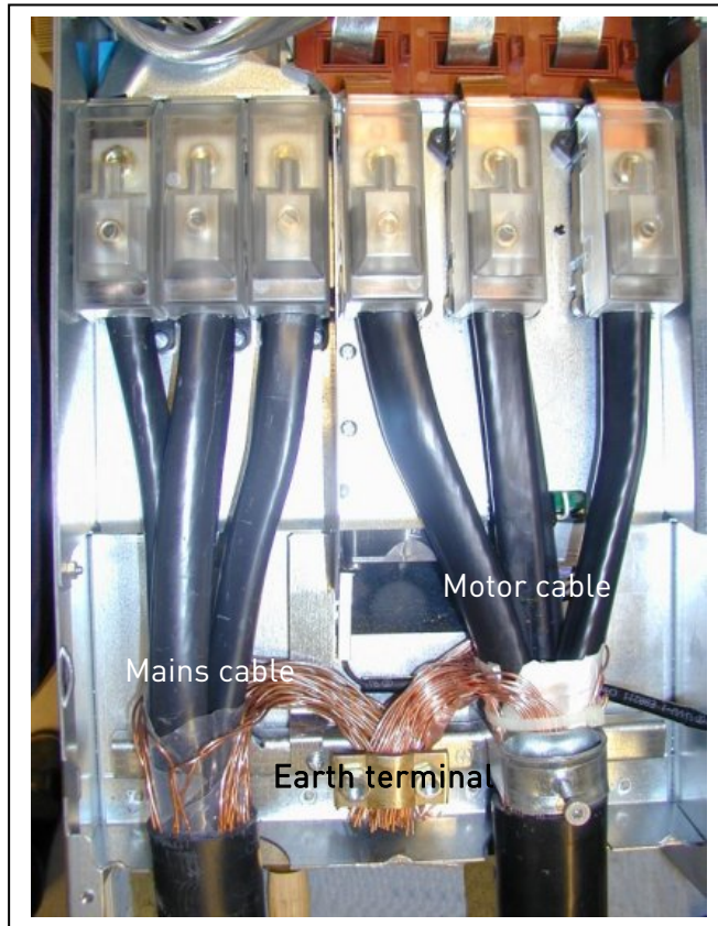
Figure 6-17. Cable installation in Vacon NXS/P, FR8
